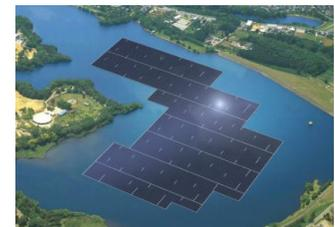
The floating arrays have many assets. They help keep water from evaporating, making the technology attractive in drought-plagued areas, and restrict algae blooms. And they are more efficient than land-based panels, because water cools the panels. The panels are specially coated to prevent corrosion, and set on a tracking system that moves them to maximize sunlight during the course of a day.
